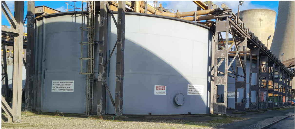
Plate 7.1 - Example of an Existing Tank
