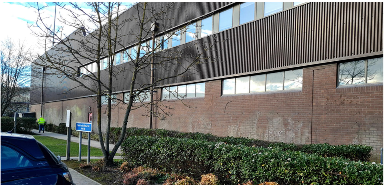
Plate 7.2 - Example of an Existing Building
